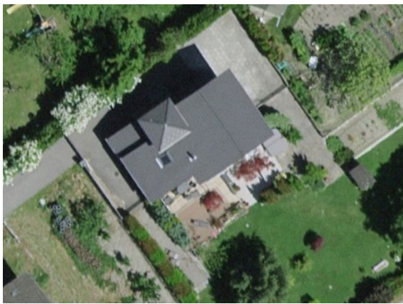
3 – Habitation, Le Belluart 4, Martigny.
