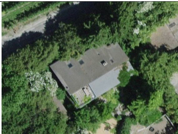
15 – Habitation, Le Belluart 6, Martigny.
