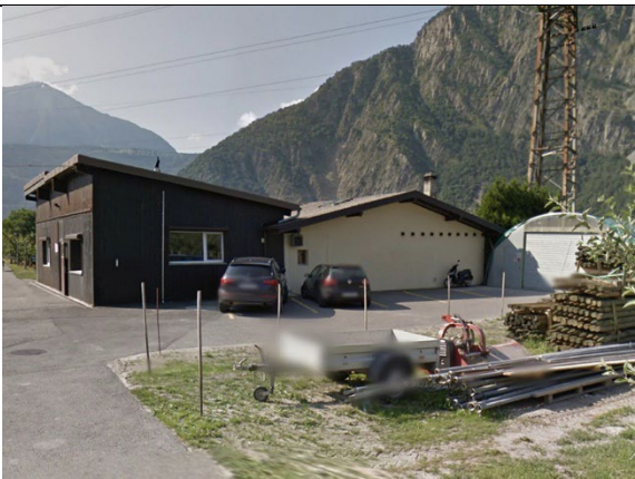
12 – Habitation, Le Belluart 3, Martigny.
